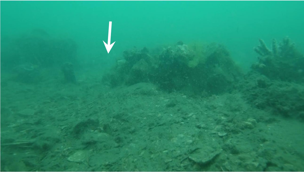
Figure 7. Photo taken from an underwater drone video showing poor condition of a patch reef deployed in 2017 which has had numerous besser fence blocks removed (arrow) and the shell knocked flat by anchor damage.
