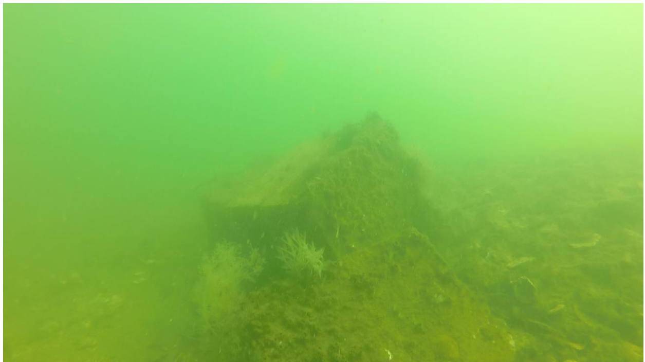
Figure 4. Anchor damage was evident on the besser block fence of the southern reef (#18). Given the increased size and weight of the fence modules used for the December 2018 deployments, this damage must have been done by a large boat powering a stuck anchor off the reef after ignoring signage and advice not to anchor in the area.
